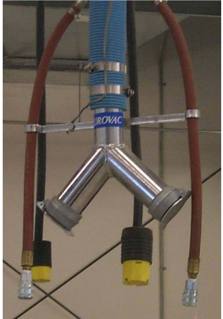
Central Dust Collection Work Bay Drop
