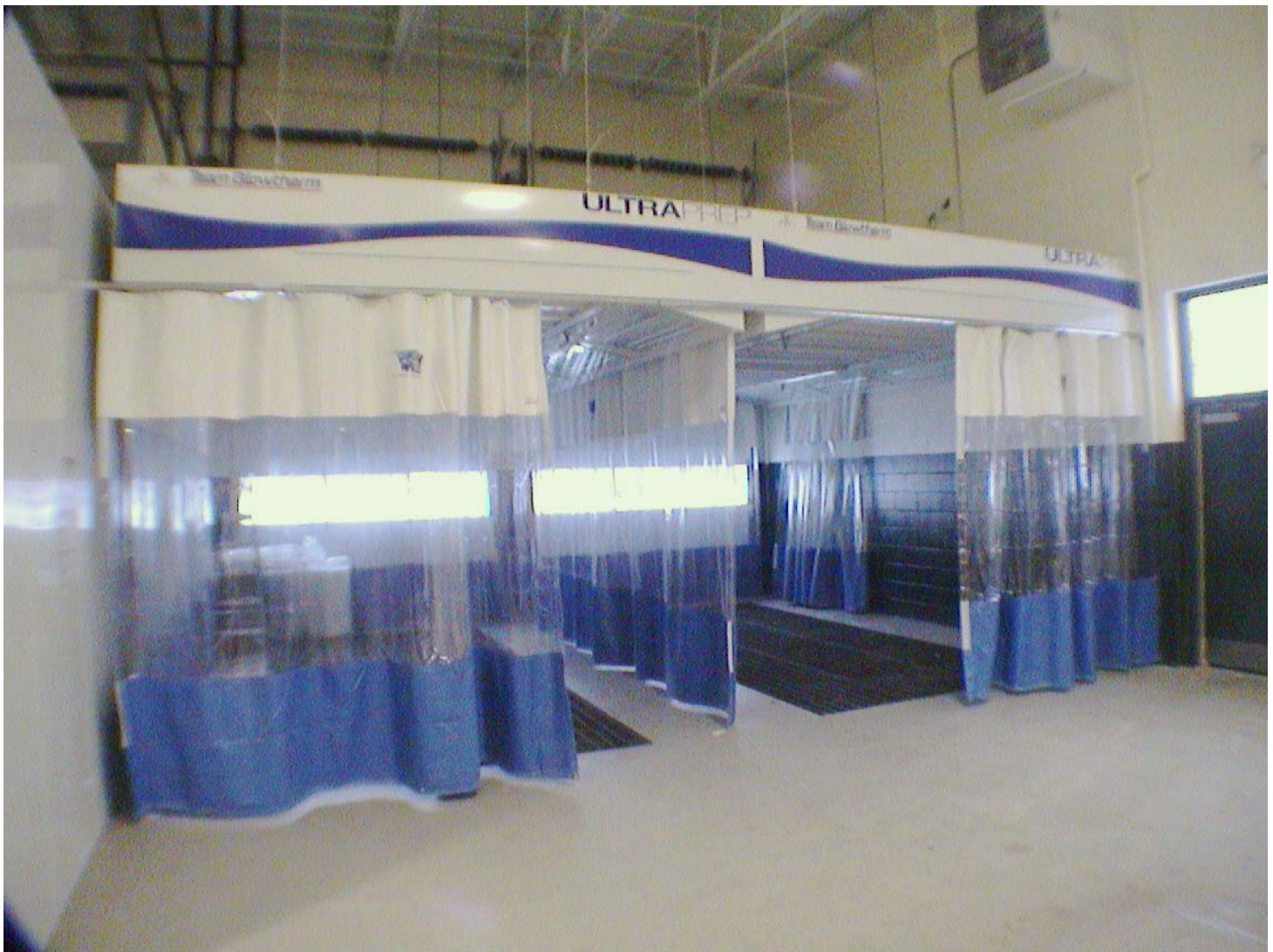
Drive Thru Limited Finishing Workstation with outside Air Replacement Unit
