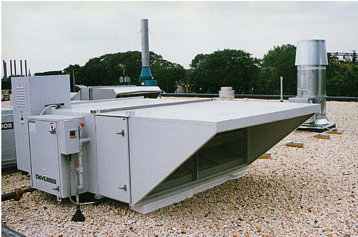
Roof Mounted Air Replacement Unit
