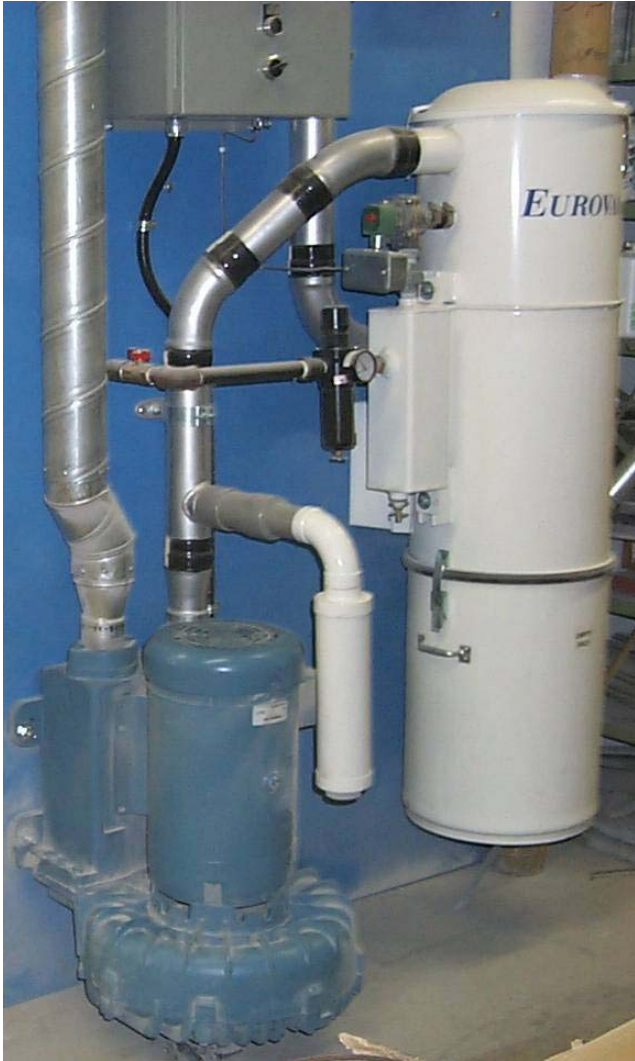
Central Dust Collection System Collector
