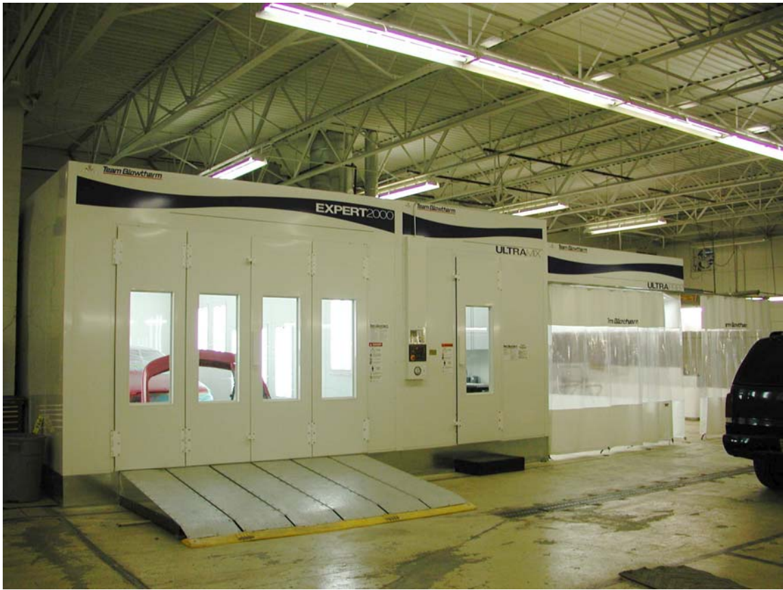
Raised Platform Spray Booth with attached Paint Mix Room
